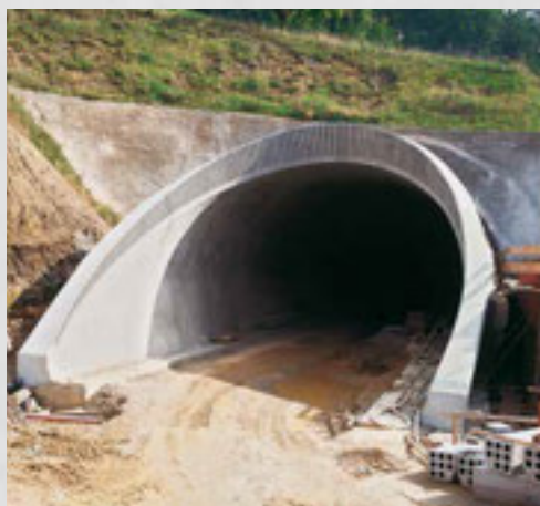
Tunnel Sommerberg, Hausach, Germania
