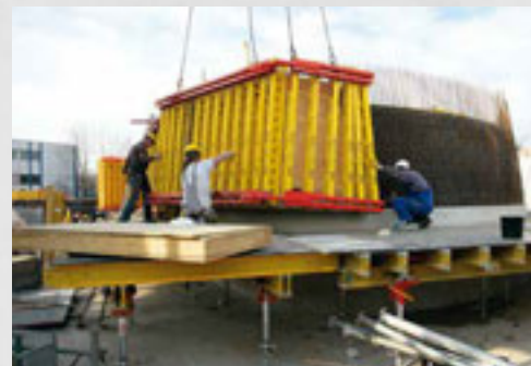
Messa in opera
