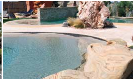
PISCINE SWIMMING POOLS
