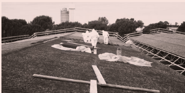
Asbestos removal
