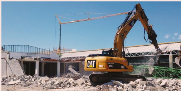
Demolition of old premises
