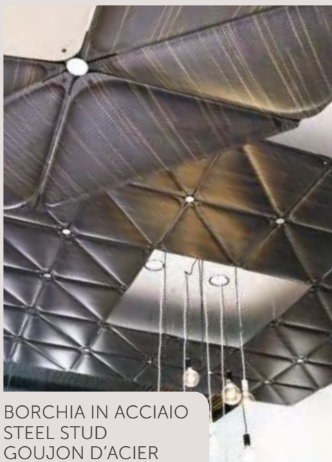
RIVESTIMENTO IN LEGNO MICROFORATO MICRO-PERFORATED WOOD VENEERING REVÊTEMENT EN PLACAGE BOIS MICROPERFORÉ
