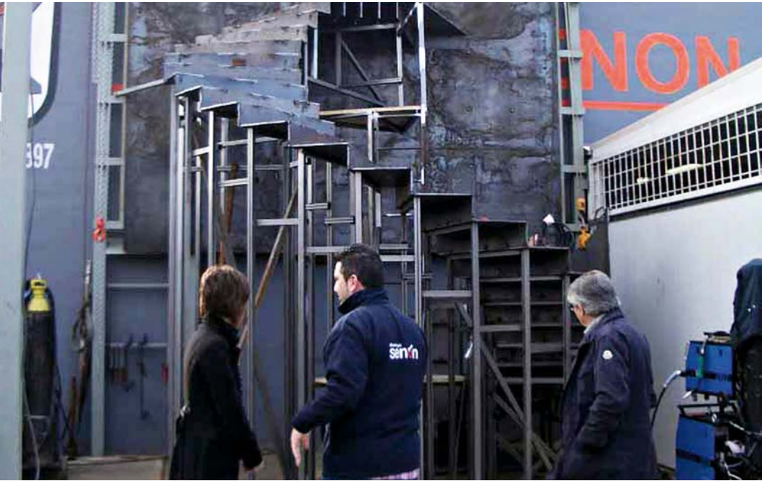
Domingo Senón: Spiral staircase construction
