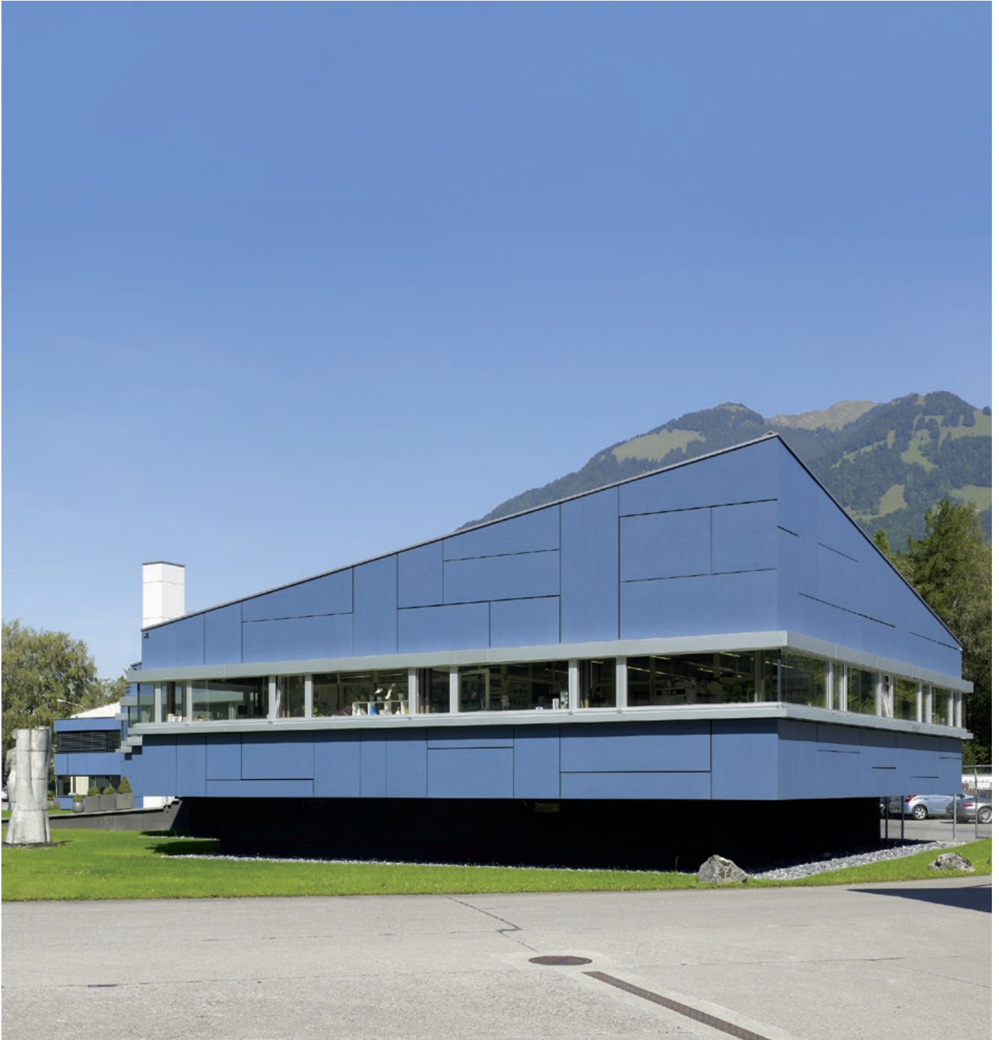
SWITZERLAND Office Building, Niederurnen
