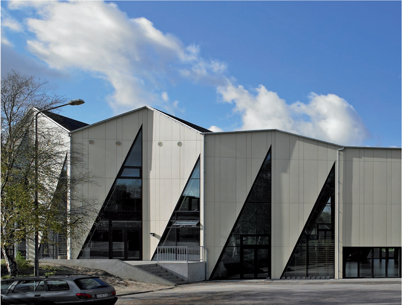
DENMARK Sports Hall Kibaek Krydsfelt, Kibaek
