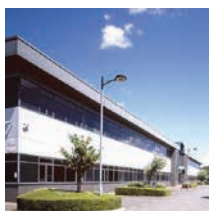
Redhill Data Centre, Redhill, Great Britain.
