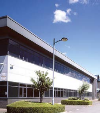
Redhill Data Centre, Redhill, Great Britain.
