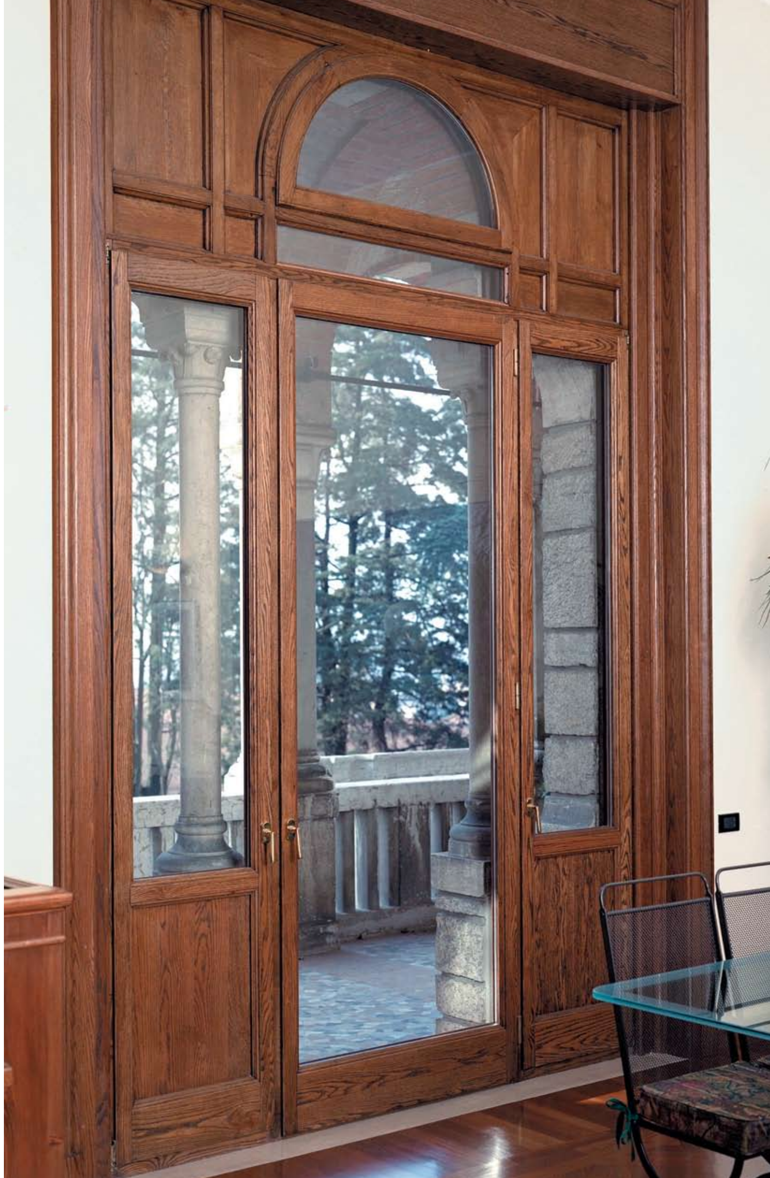
Serramento SC 70 in rovere (sopraluce restaurato) SC 70: entrance door in Oak (transom restored)
