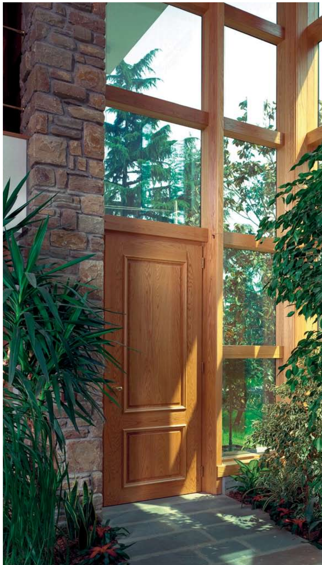
Wood-glass: facciata continua strutturale in rovere e vetro Wood-glass: structural curtain wall made of Oak
