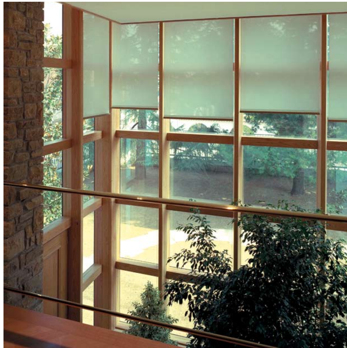
Wood-glass: facciata continua strutturale in rovere e vetro Wood-glass: structural curtain wall made of Oak
