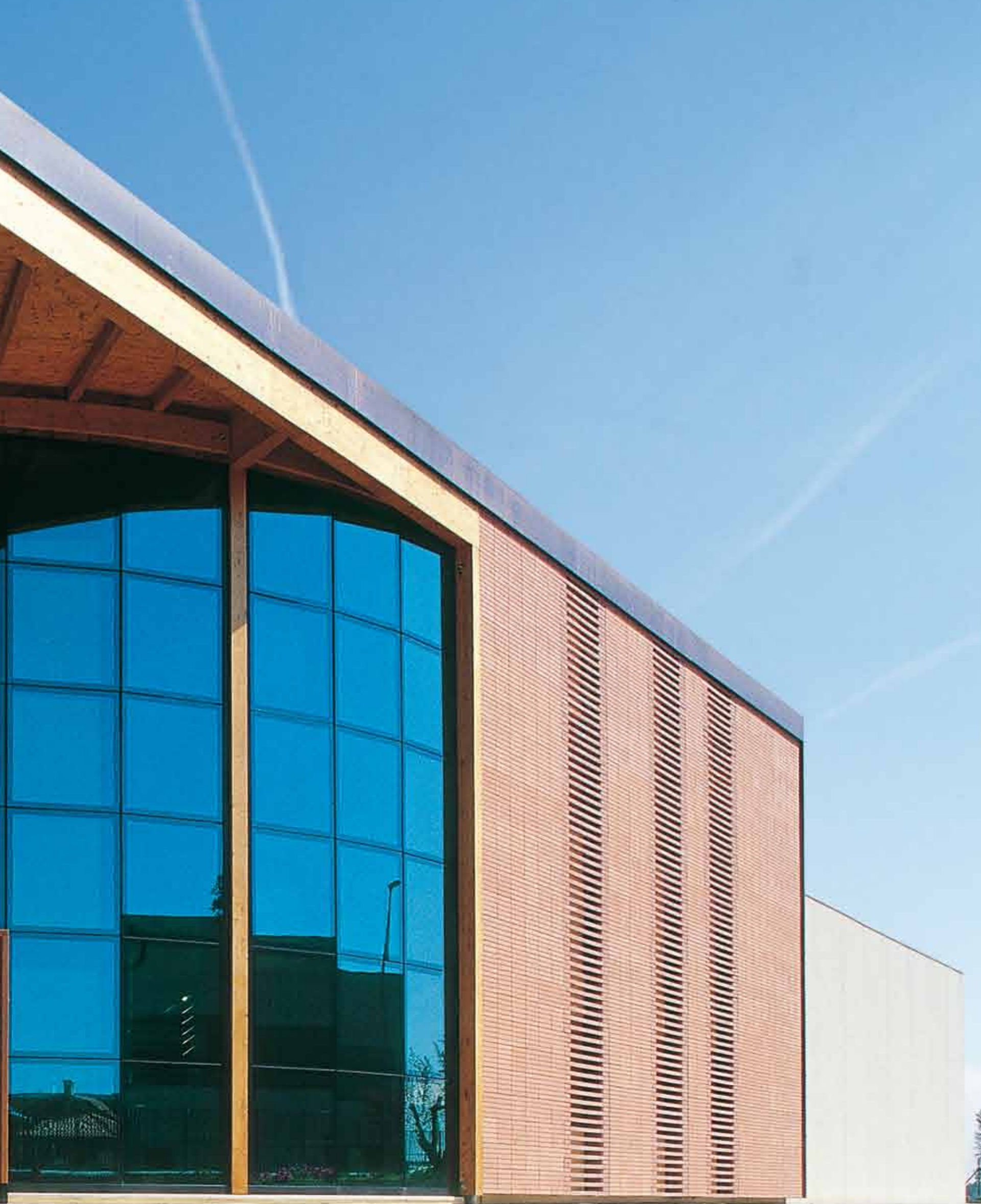
Wood-glass (facciata continua in legno) Wood-glass (wooden curtain-wall)
