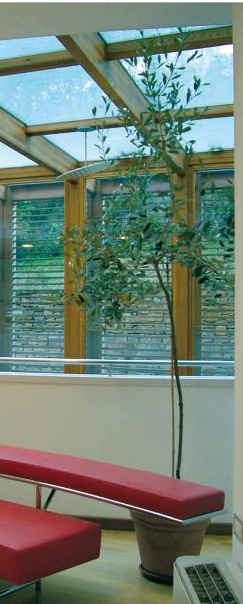
Tetto Cielo in legno e vetro Roof structure in wood and glass
