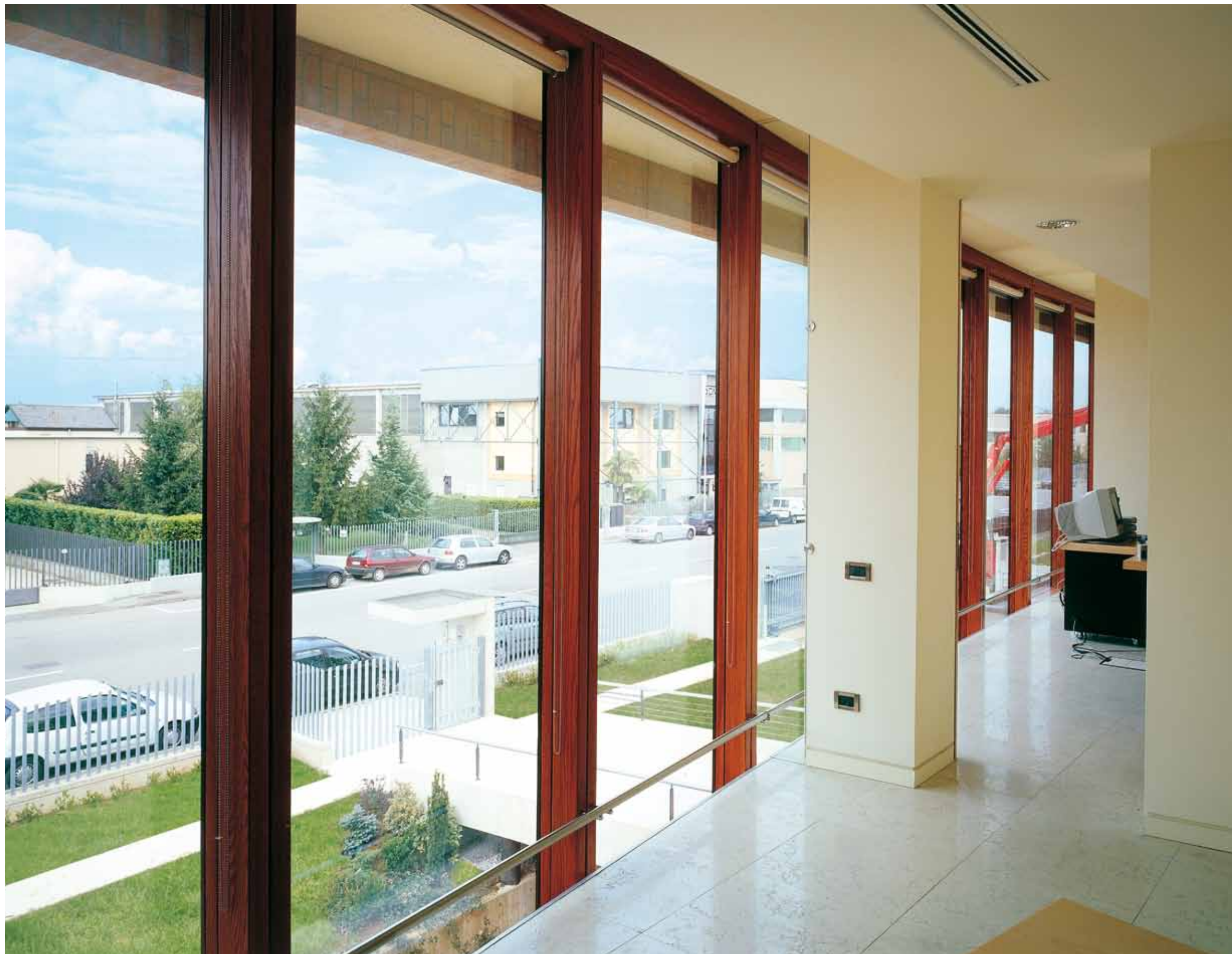
Wood-glass (facciata continua in legno) - Wood-glass (wooden curtain-wall)
