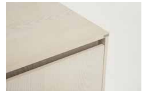
Distance between door and frame for ventilation.
