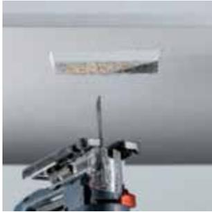
*Take measurements and cut the plasterboard*
