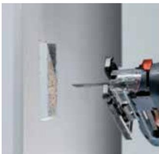
*Take measurements and cut the plasterboard*
