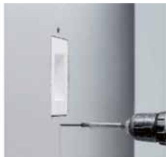
*Screw the spot together with the plasterboard*
