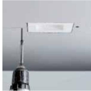
*Screw the spot together with the plasterboard*
