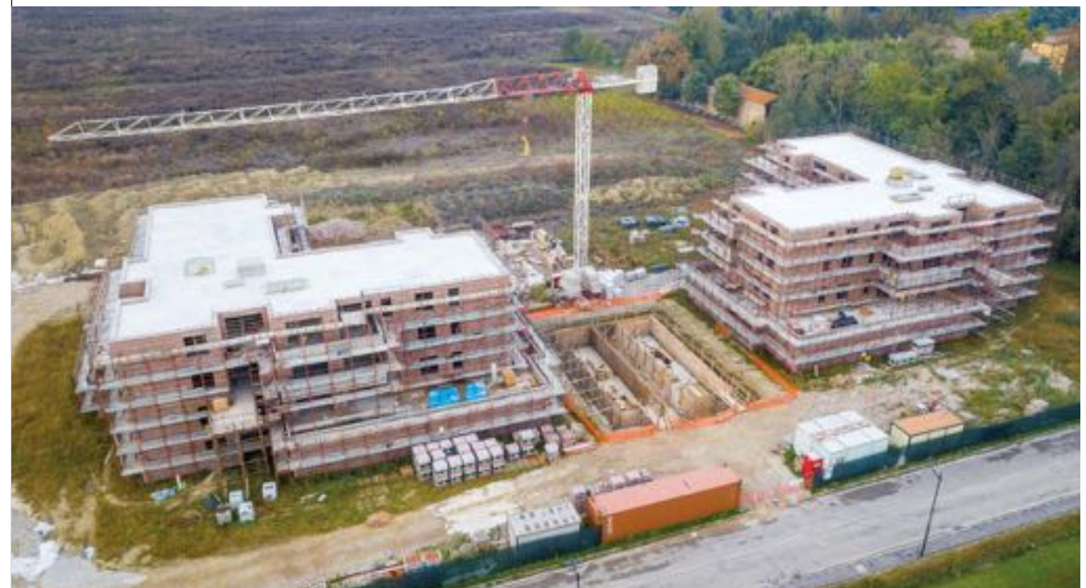
Intervento Social Housing 40 alloggi a Molinella (BO) - 2020
