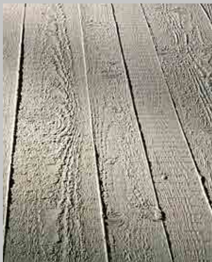
CONCRETE TIMBER FORMWORK √ bordo abbinato ABS 25x1 mm
