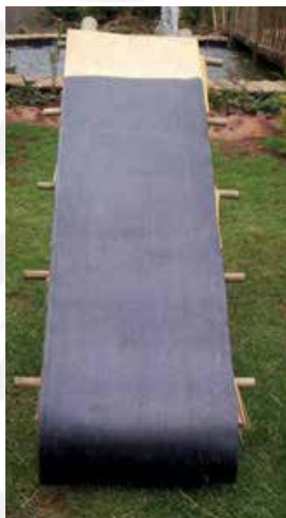
4 a fase: Posizionamento guaina isolante 4th step: Waterproofing material is stapled
